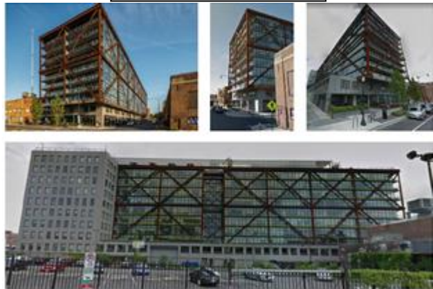
Views of the Existing Building
